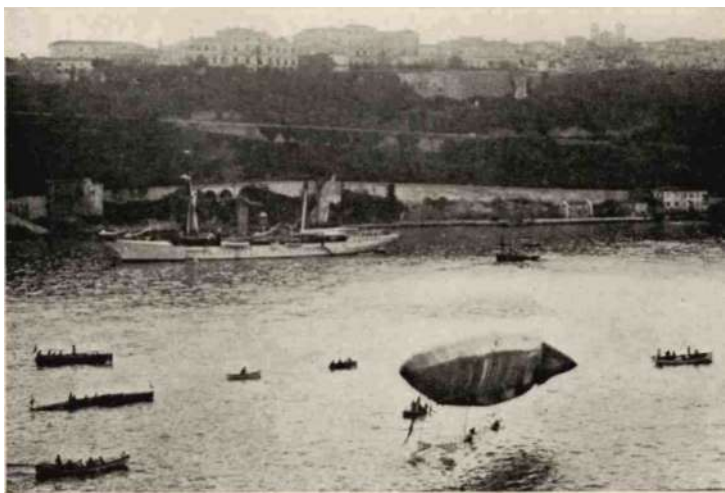
Phase D — before final collapse Accident, February 14, 1902
