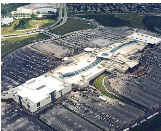
Figura 5.33 Mall At Millenia - vista aérea. Fonte: www.thedibb.co.uk/forums/ , 14 fev. 2005.
