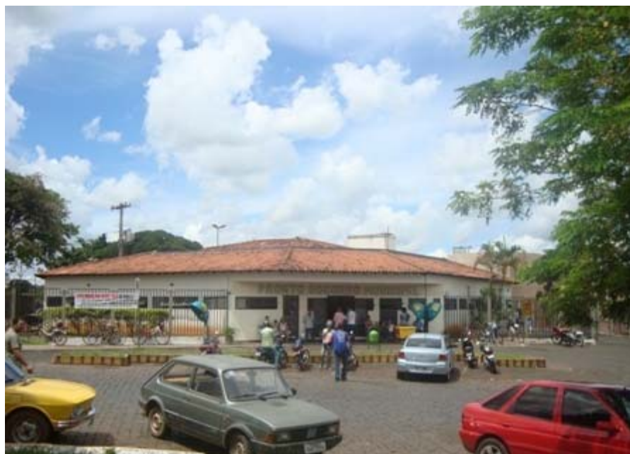
Foto 42 - Araguari (MG): Pronto Socorro Municipal (2009)
