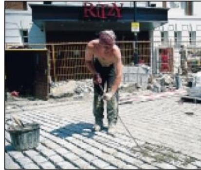
London's lost heritage. Expensive high quality setted surfaces are common under later layers of tarmac. Old concealed setted surfaces can be exposed easily and restored to provide effective traffic calming
