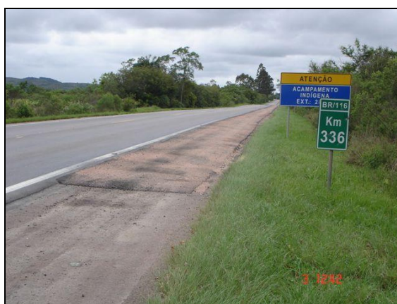
Figura 60 – Trecho 01, BR 116, Km 336
