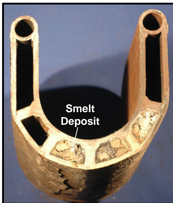
Figure 13. Crossed section of spout #5, showing smelt deposits locking cooling water passage.
