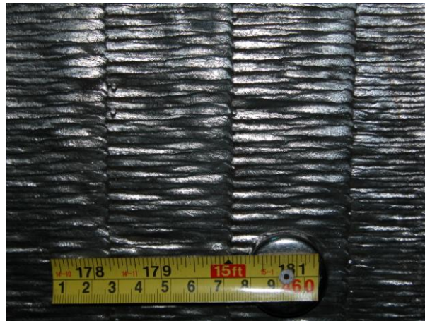
Figura 3.25: weld overlay vertical acabado (Wensley, 2004).
