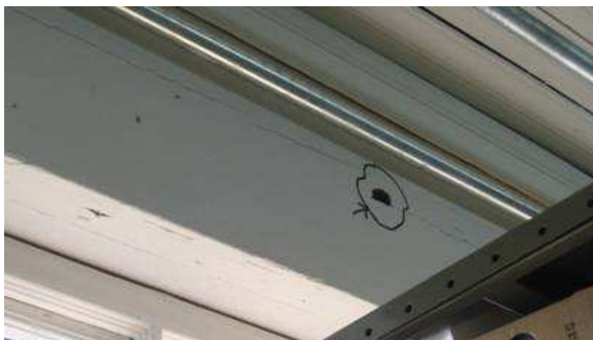
FIGURA 4.16 – Viga principal perimetral externa.
