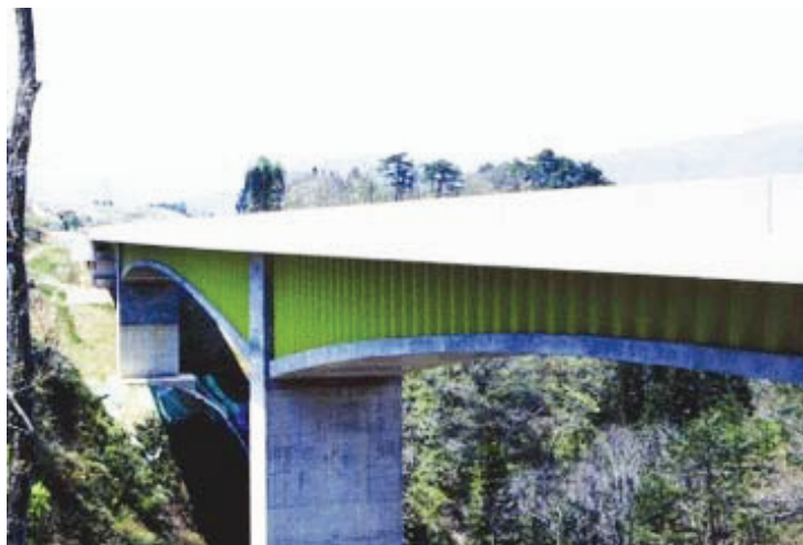
FIGURA 1.7 - Ponte Hondani [PLAIS (2005)]
