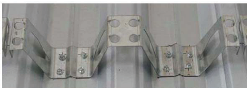
FIGURA 2.3 – Conector Stripcon ou Ribcon [MOTAK & MACHACEK (2004)]
