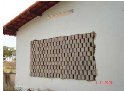
Figure 12: Photo of the block type 1 seated in front separated 5 cm
