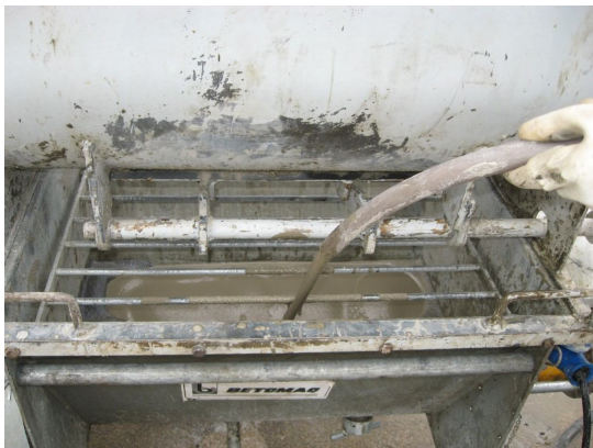
(c) Graute na betoneira
