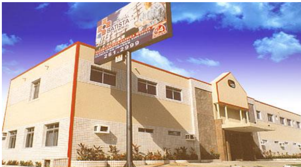
Figura 3: Hospital Batista Memorial – Fortaleza-CE
