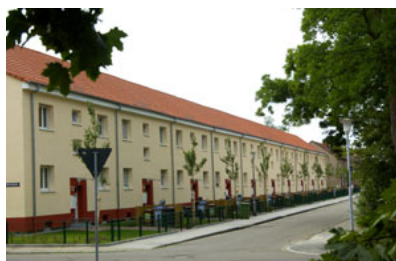
Figura 49: Garden City Rehabilitated Apartment Complex
