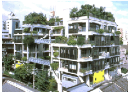
Figura 95: NEXT21 experimental condominium
