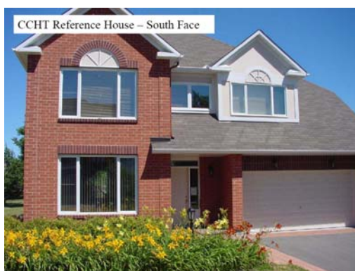
Figura 77: Canadian Centre for Housing Technology
