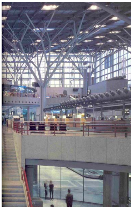
Figura 3.58 – Obra: Stuttgart I. Airport
