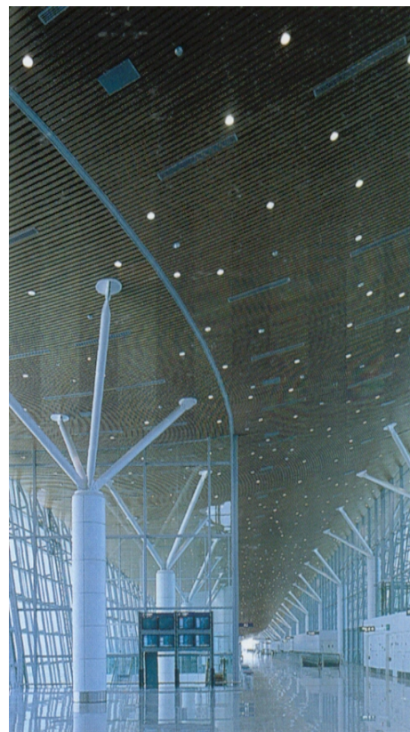
Figura 3.57 – Obra: Kuala Lumpur I Airport
