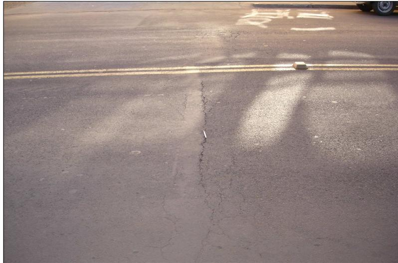
Figura 42 – Trincamento Transversal
