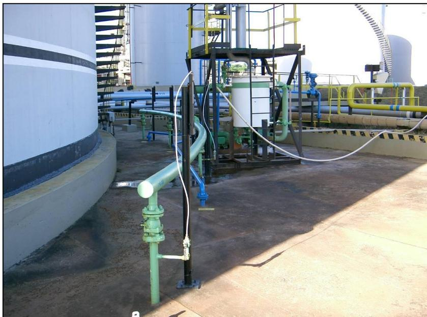
Figura 17 - Sistema piloto air sparging/soil vapor extraction
