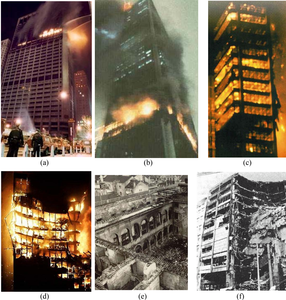
Figura 2.14 - (a) Meridian Plaza na Filadélfia - EUA, em 1991, (b) Edifício do Firts Interstate Bank em 1988; (c) Edifício da CESP, em São Paulo — 1987; (d) Torre Windsor, Madrid, 2005, (e) Museu Colonial de Lisboa; (f) Edifício Katrantzos Sport, em Atenas, na Grécia — 1987; fontes (a) http://911research.wtc7.net/talks/b7/history.html , (b) http://911research.wtc7.net/cache/wtc/analysis/compare/lafire_firstinterstate.htm , (c) e (d) http://www.lmc.ep.usp.br/people/valdir/?page_id=16 , (e) http://www.triplov.com/politecnica/fotos_museu_bocage/pages/a_incendio.htm e (f) http://www.fpemag.com/archives/article.asp?issue_id=27&i=153 .
