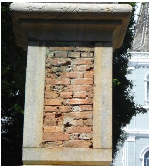
Figura 12: Placa frontal (Foto: Giliard Prado, 2007)
