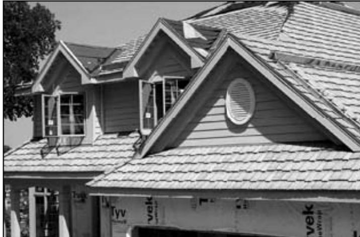
Figura 4: Telhado de WPC (Caulfield, 2005)
