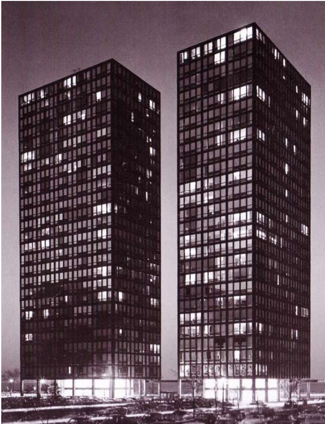
Lake Shore Drive Apartments, Chicago, 1952.
