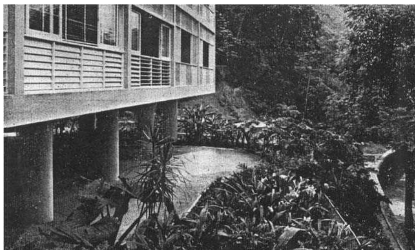
Fig.155: Fachada principal e entrada social
