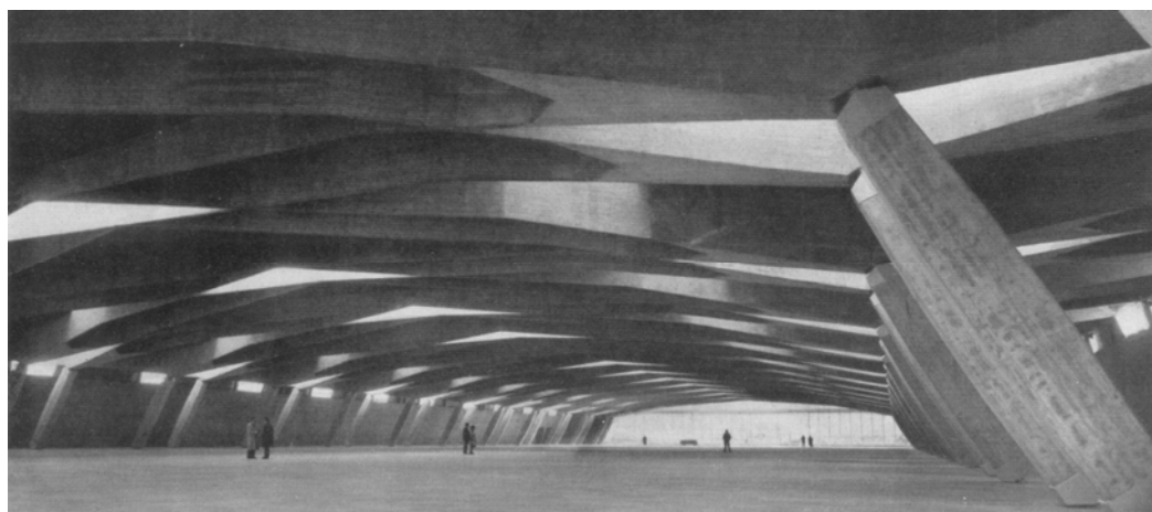
Fig.744: Vista do interior
