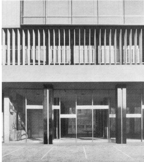
Fig.367: Entrada principal - hall
