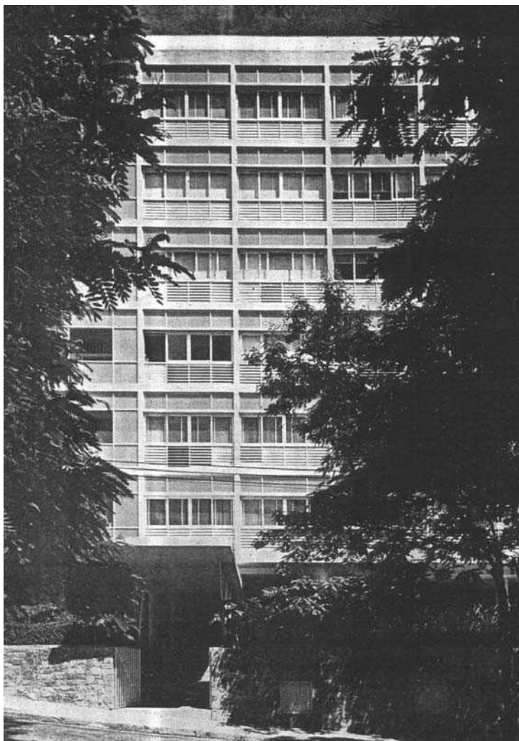
Fig.154: Fachada principal e entrada social
