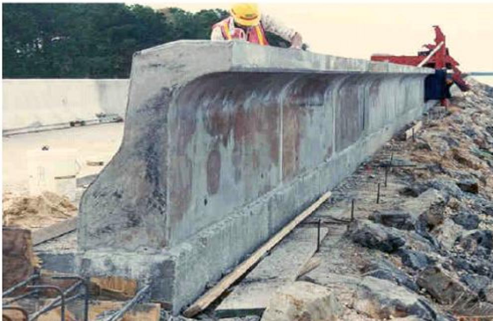
Figura 2.7 – Muro de parapeito curvo (U.S. Army Corps of Engineers, 2004).
