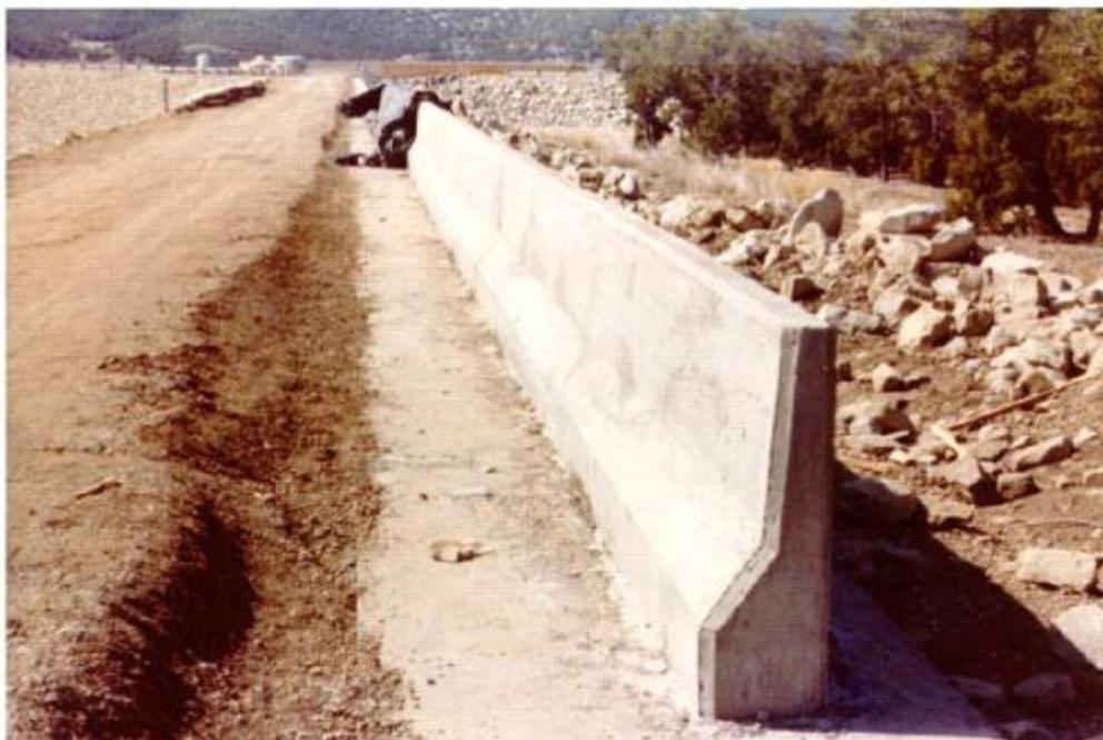
Figura 2.8 – Muro de parapeito convencional (U.S. Army Corps of Engineers, 2004).
