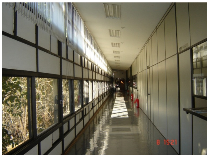
Figura 53 – Interior do Bloco E1 – 2007
