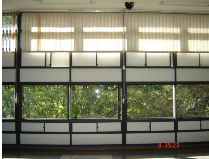
Figura 54 – Interior do Bloco E1 – 2007
