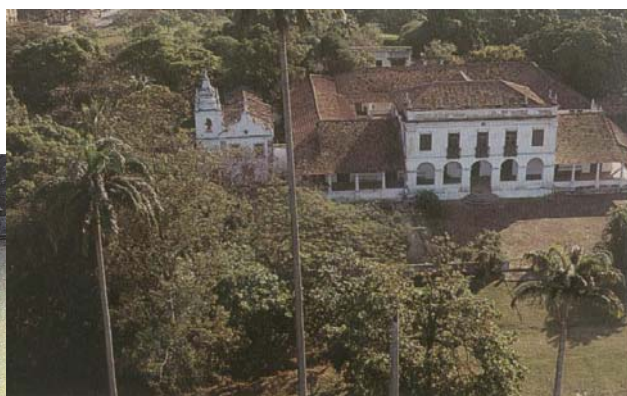
II.59. Vista geral
