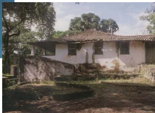
II.58. Rampa externa lateral
