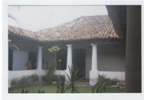
II.36. patio interno
