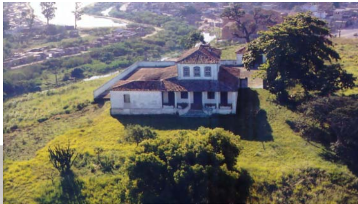
II.50. Vista geral
