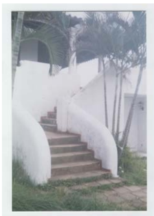
II.46. escada externa
