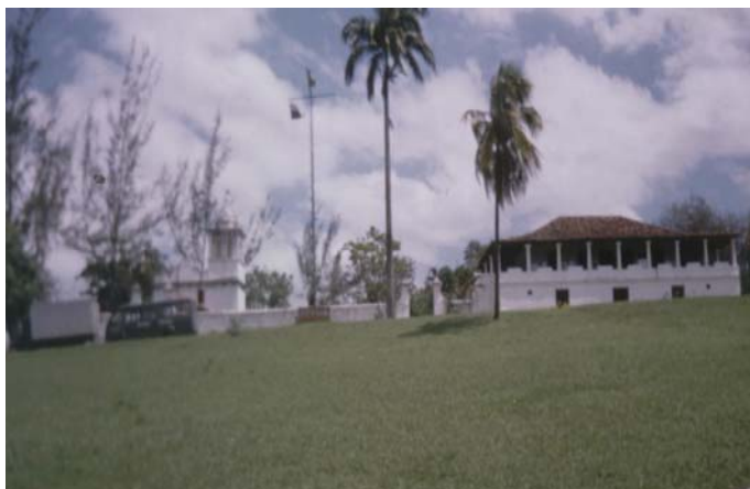
II.45. Vista geral
