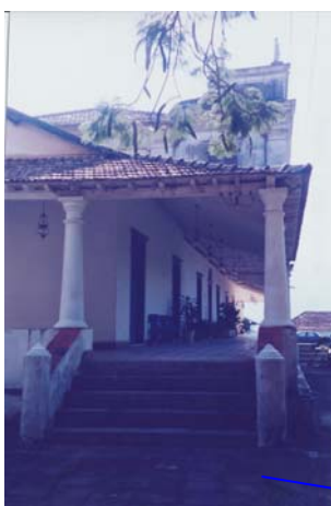
II.62. Escada externa
