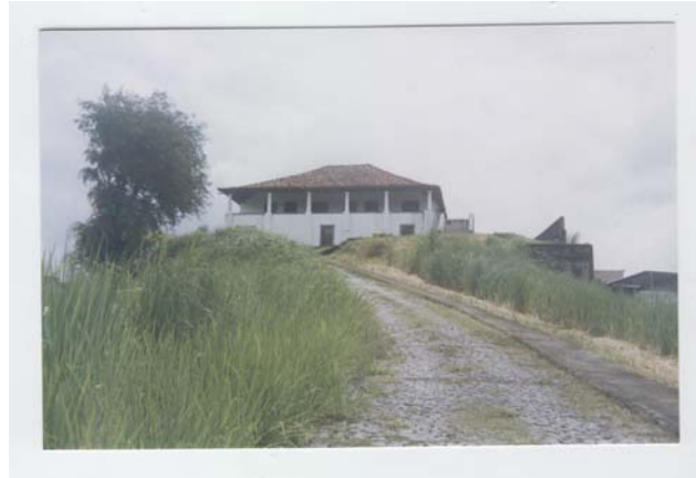
II.40. Vista geral
