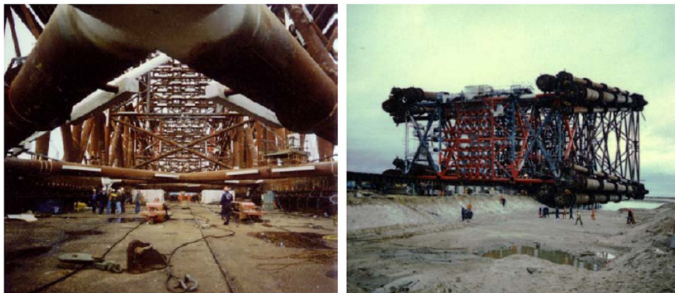
Figure 2.7: Photographs of the North West Hutton Jacket
