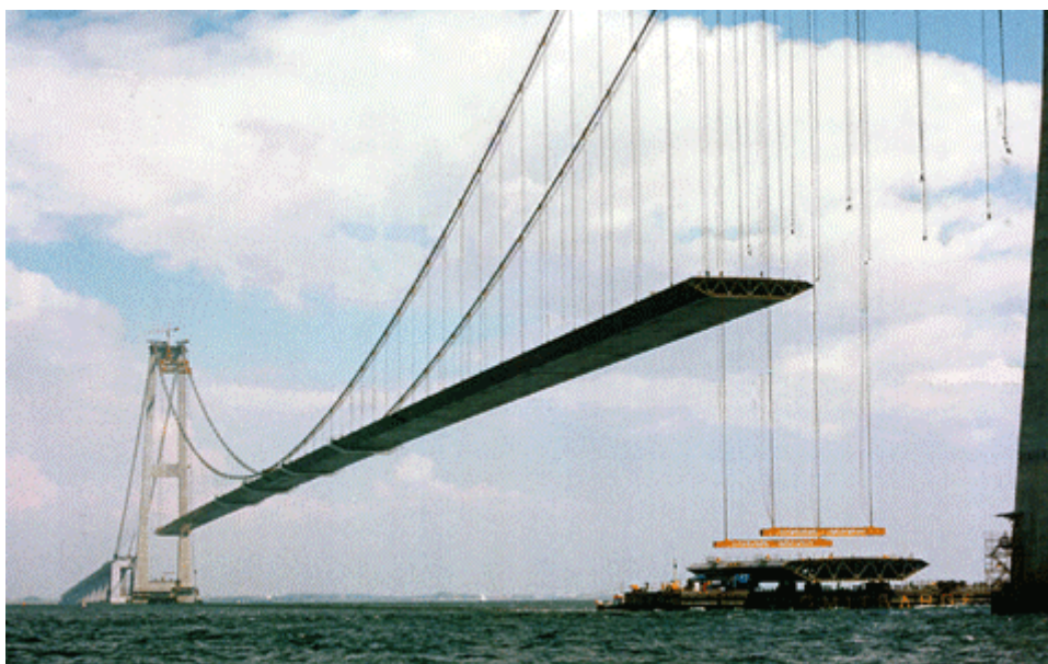
Fig. 2.17 – Ponte Great Belt East – Dinamarca.
