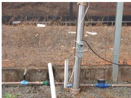
Figura 8A – Reator ultravioleta
