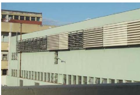
FIGURA 127 – Vista externa - bloco com *brise-soleils*
